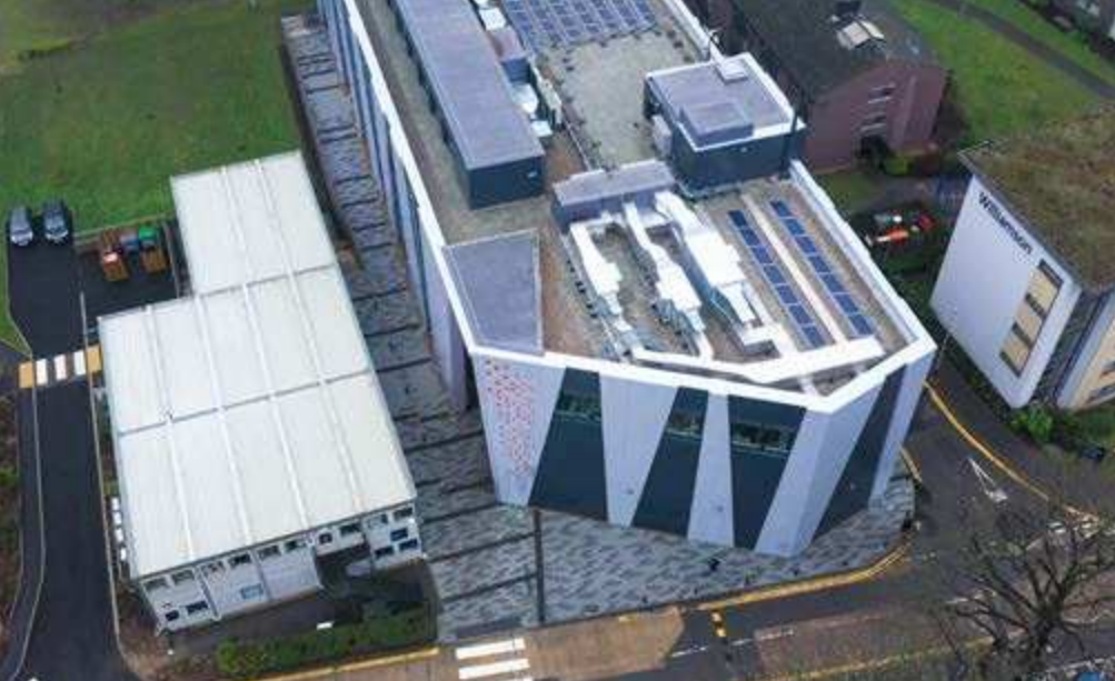
The sustainable energy rooftop lab at Shilling Building
